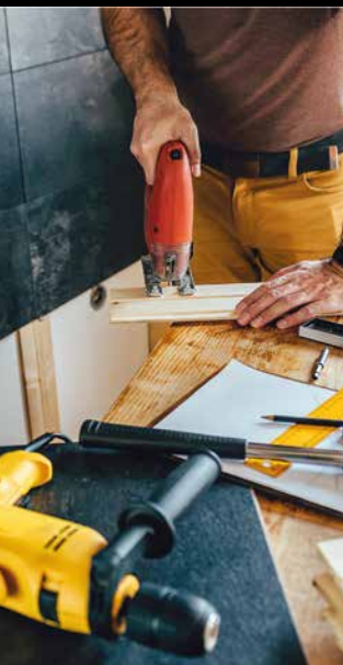
Construction sites / renovations
